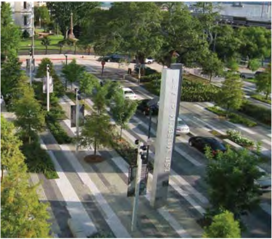
ENHANCED VEHICULAR PAVING AT MOTORCOURTS 6"x24"x4" PAVERS BY STEPSTONE OR SIMILAR
