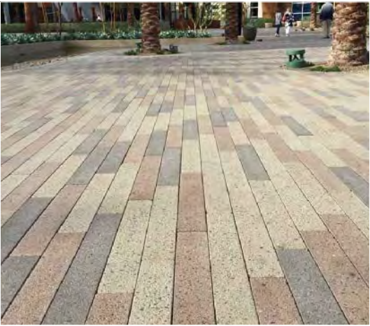
DECORATIVE PAVING AT OUTDOOR CAFE AREA 3"x24"x4" PAVERS BY STEPSTONE OR SIMILAR
